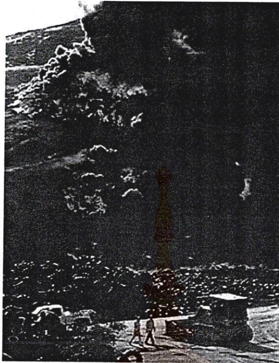
Figure 2. 2 Tyre fire in Stanislasu Company, California in 1999 (Reschner, 2008)
